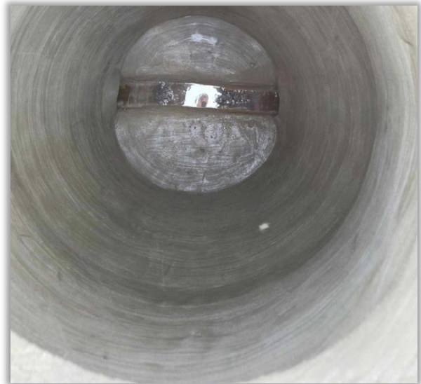
The City contracted with SAK for "cured-in-place" sewer rehabilitation and manhole rehabilitation. This prevents further breakdown of sewer line and manholes through a relining process which provides greater structural integrity.
